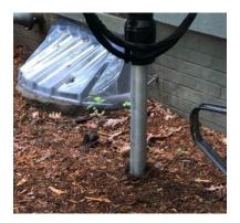
Should churning or auguring occur without immediate correction, the screw should be removed and repositioned. If using the same hole is required, 3/8" "chip" gravel can be poured into the hole to re-establish the load-ability following the installation procedures described above. A maximum of 20 RPMs is advised and only with a mechanical driver capable of enough crowd to advance the screw as described above.
